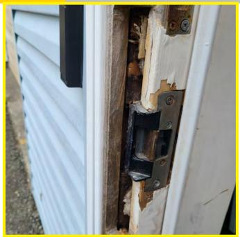
The photo above shows a clear example of building envelope failure at the rear entry door jamb. Rot and deterioration is clearly present and likely is also present within the wall assemblies. The section of rot lessens the security level of this entry point.
