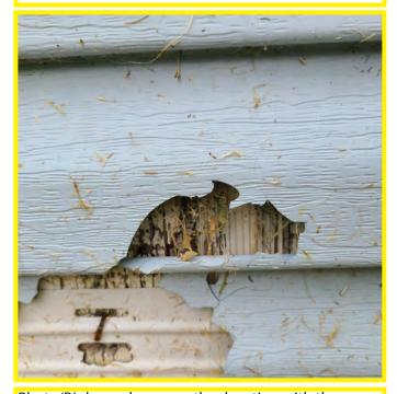
Photo 'B' above shows another location with the same issues as seen in photo 'A' to the left. The plywood wall sheathing is exposed and no building paper or weather barrier is seen which is a major building envelope assembly issue.
