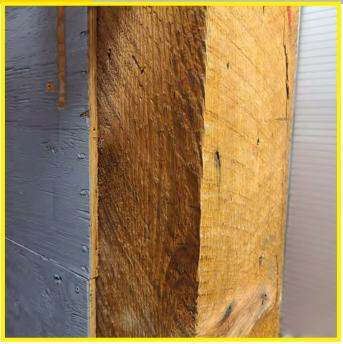
The photo above shows a close up look at the roughsawn columns and what is assumed to be a shear wall nailing pattern at the edges of the plywood sheathing. The structural adequacy of the columns and acceptability of the nailing cannot be confirmed.
