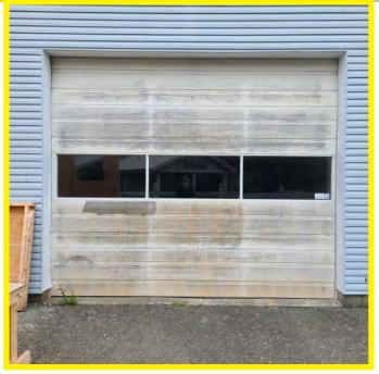
Photo above shows rear overhead door has surpassed its product life cycle. This overhead door may be an acceptable size if used only for access and egress of small equipment.
