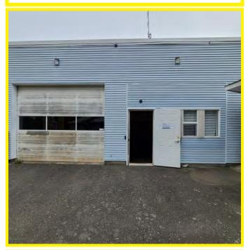
The photo above shows the overall facade deterioration and inadequate site lighting. Lighting should be upgrade to LED for energy efficiency. Windows and doors should be replaced for improved energy efficiency. No door panic hardware for exiting.
