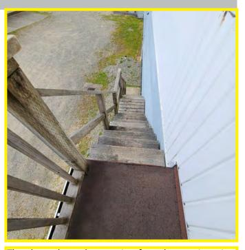
The photo above shows a view from the exterior exit stair landing to the ground. The landing surface is deteriorating and narrow. The hand rail is not of an acceptable design. NOT TO CODE/ unsafe for use.
