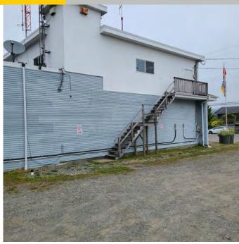
The photo above shows the patchwork of cladding materials and the only second level emergency exit staircase. Consistent lot deterioration is shown in this area as well.
