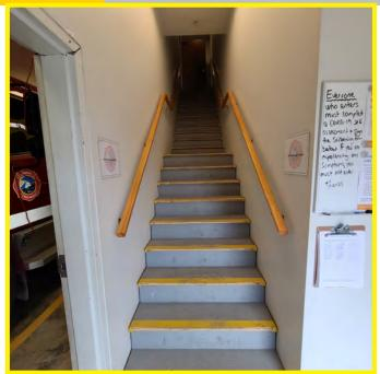
The photo above highlights the stair and handrail issues. The stair treads do have proper nosing but have a steep rise and run and inadequate headroom as required by code. The door frame appears to be poorly installed or unfinished.
