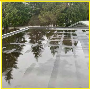
The photo above shows the general condition of the roof. The roof system is inadequately sloped causing water ponding during the fall and winter months. It is clear that the roof requires replacement.
