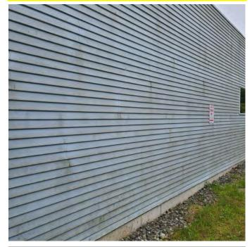
Photo above shows vinyl exterior wall cladding. It is obvious that the vinyl cladding has exceeded its product life cycle and needs to be replaced. Immediate maintenance is required. Significant signs of weathering.
