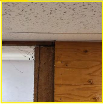
The photo above shows a close up look at one of the interior partition walls. This wall is assumed to be a structural shear wall supporting the floor above. The connections do not appear to be seismically sound.
