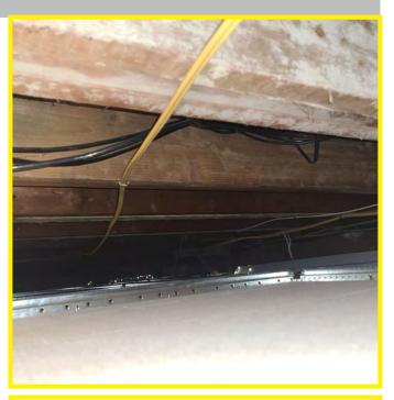
The photo above shows a look above the apparatus bays acoustic ceiling tile finish. The t-bar does not appear to be seismically fastened to the underside of structure. No fire rating is observed. The structure appears to just be dimensionally wood framed.
