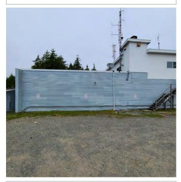
The photo above shows an exterior view of the lower level administrative building components. No parking is available along this facade. The flat roof drains through scuppers and downspouts as shown in the photo above.
