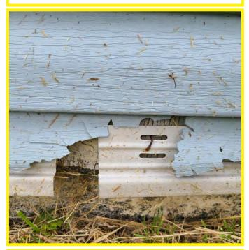
Photo 'A' above shows one example of complete building envelope failure. The vinyl cladding has long passed its product life cycle and is brittle and crumbling. This residential style product is combustible and not suitable for this application.
