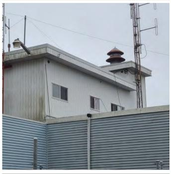
Photo above shows rear of second storage. It is obvious that the building envelope has failed. Roof scuppers require replacement. Exterior mounted equipment needs relocation and proper mounting.
