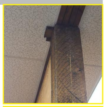
The photo above shows an exposed 4-ply built-up wood beam supporting the floor above. It is assumed these members are continuous over the column support. Proper structural fastening or metal brackets appear completely absent. Shimming is wedged.
