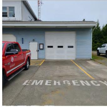
Added apparatus bay. Overhead doors are smaller than industry standard. Needs 12'Wx14'H min. size.
