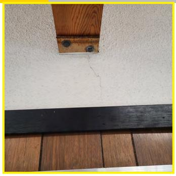
The photo above shows drywall cracking below the glulam beam which indicates building movement and/ or settlement.
