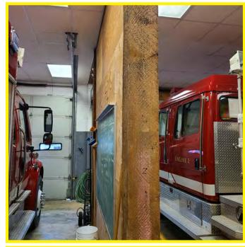
The photo above shows a dividing partition wall between the main truck bays. This wall is comprised of rough-sawn timber columns and plywood sheathing. This wall is assumed to be a structural element. No fire rating protects these elements.
