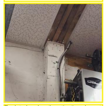
The photo above shows the continuation and support of the structural floor beam member terminating at the front wall location. The size of column is unknown. The column is assumed similar rough-sawn wood. Proper bearing? Lack of fastening. NON-SEISMIC.
