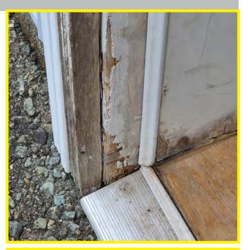
The photo above shows a rotting rear door jamb and interior base of wall near the sill. It is clear that proper door installation details were not followed allowing water leakage into the building envelope. A commercial type door should have been used.
