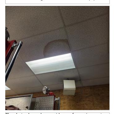
The photo above shows evidence of a previous water leak and subsequent water damage to the ceiling finish. It is assumed this did not cause any structural damage. A small unit heater is hung from the ceiling space and does not appear adequate for the space.
