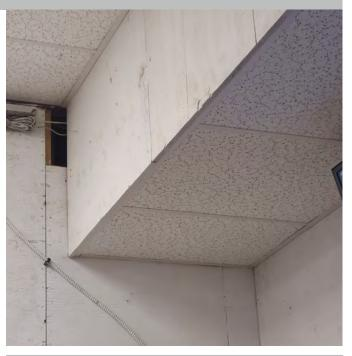
The photo above shows the poor patchwork condition of the interior wall 'finishes' and surface mounted electrical. No fire rated material is observed around bulkhead areas.
