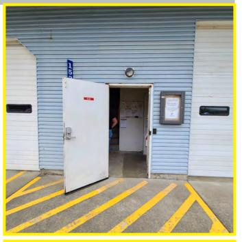
The photo above shows inadequate main entry lighting. The main entrance is not suitable for public access. Emergency egress (panic) hardware is not present.
