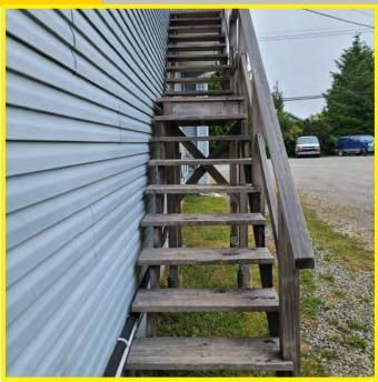
The photo above shows exterior mounted electrical conduit along the vinyl clad wall face. This conduit should be protected. The stairs show significant signs of weathering. The steps and railing are not to building code standards and are loose.
