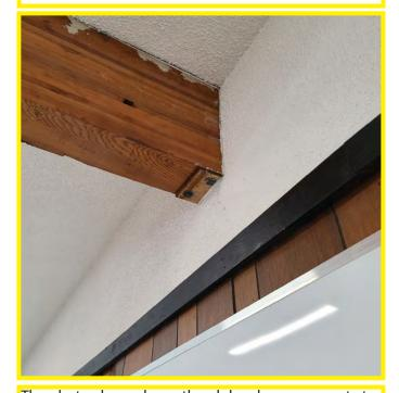
The photo above shows the glulam beam support at the front exterior wall. The beam is fastened to a metal bracket. The integrity and adequacy of this connection cannot be confirmed. It does not appear seismically sound.
