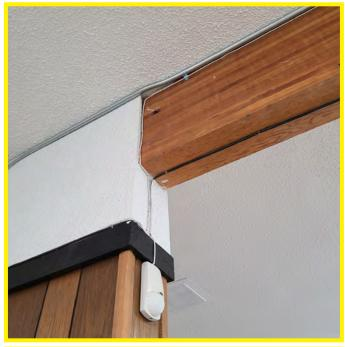
The following photos show elements of the supporting roof structure. A single exposed glulam beam is observed. The bearing and support column is hidden in the wall and cannot be confirmed adequate.
