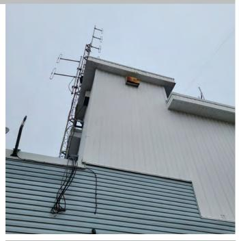
The photo above shows poorly sealed wall penetrations and cladding details. These areas are prone to weather intrusion. Building envelope leaks lead to rot, mold growth, health hazards, and energy performance loss.
