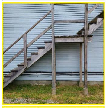
The photo above shows construction of exterior stairs. The staircase is not built to code and is inadequate for use as an emergency exit.
