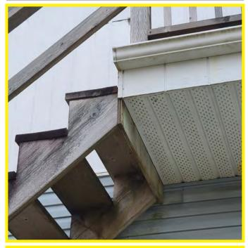
The photo above shows that the stair is not structurally safe. The stairs are deteriorating and should not be used. A small exterior gutter is observed.
