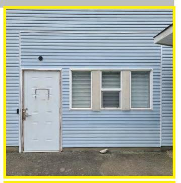
Photo above shows patchwork to building envelope and inadequate window and door details. It is assumed that the building envelope has completely failed and no long keeps out water from the wall assembly. Windows are old and past product life cycle.
