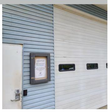
The photo above shows the main entry door and apparatus bay overhead doors. The doors and front facade have consistent wear and signs of weathering as the rest of the building. While the style of overhead doors are acceptable, they are too small.
