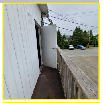
The photo above shows a number of building code and life safety concerns. This exit stair is unsafe for use. The railing is not secure, the door does not open fully, there is no door panic hardware for exiting, the landing is deteriorating, the overhead power lines to the building are not placed safety or neatly, etc..
