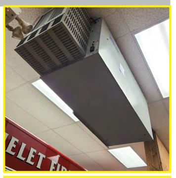
The photo above shows a single air scrubber unit centrally hung over the main apparatus bays. Efficacy cannot or proper operation cannot be confirmed to meet WCB standards with respect to controlling carbon monoxide levels from truck exhaust.
