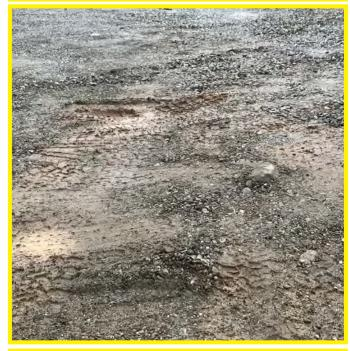
The photo above shows soft spots in the parking and training area of the site that become too soft to drive apparatus trucks over in the fall and winter months. Removal of soft areas and installation of structural fill materials is required in these areas.
