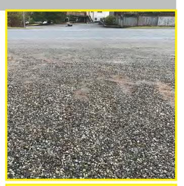
The photo above shows that although most of the site appears generally stable during warm dry months, poor soils conditions and soft spots become visible during the fall and winter months. Geotechnical investigation should be conducted.
