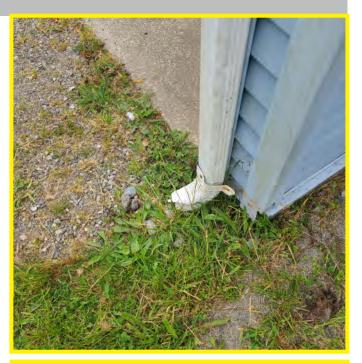
Photo above shows downspouts draining to surface. No splash pads are observed to prevent ground erosion. Ground shows significant organic growth around building in 'non-landscape' areas.
