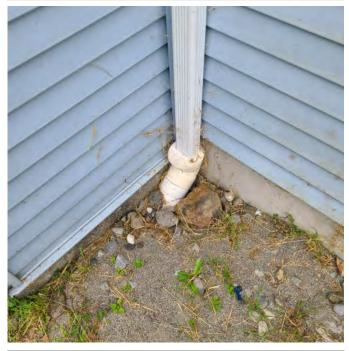
Photo above shows that a perimeter storm water management system is present. The connection appears to be shallow depth. Ground appears unstable due to erosion and organic growth.
