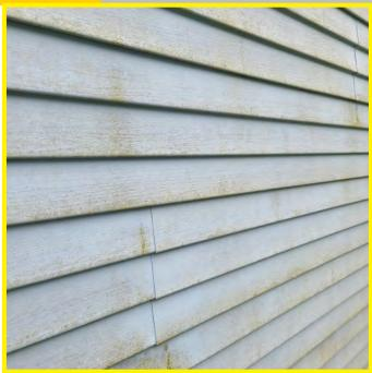
Photo above shows a close up of the exterior vinyl cladding. This material should not be used on a building of this type. Significant signs of weathering are further shown. Exterior cladding should be replaced with a non-combustible material.
