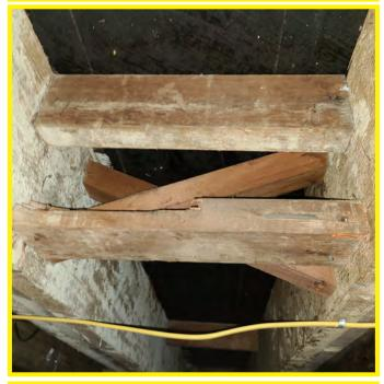
The photo above shows a closer look at the 2nd floor framing elements. These do not appear to be seismically sound. The wood is dry but it not in good condition. The wood has the appearance of used forming material. - structural details needed.
