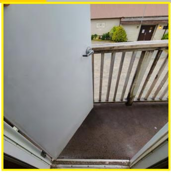
The photo above shows the second floor emergency exit stairs. The door does not have any emergency panic hardware and the door can only open approximately 75 degrees. The railing wood railing is weak and shows signs of significant weathering.
