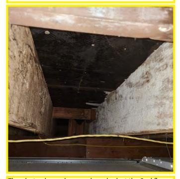
The photo above shows a closer look at the 2nd floor framing elements. Joist bracing or blocking appears to be inadequate. No fire rating is observed. Stuctural framing needs to be inspected by an engineer. Replacement and increased fastening requirements.
