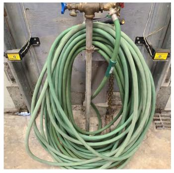
The photo above shows an interior hose bib that is used for vehicle washing. This needs to be relocated and mounted for proper storage.
