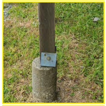
The photo above shows the stairs structural support is inadequately and improperly installed. This detail will cause eventual rot even to pressure treated wood materials. Proper installation and structural fastening is required for life safety areas.
