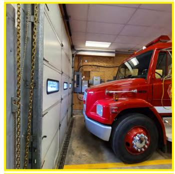
The photo above highlights a number of major issues with the existing Fire Hall that further stress the need for an A&R or new Fire Hall to be constructed: OH door/ drainage, electrical issues/ fire hazards, there is NO ROOM for an aerial truck of adequate walking rm.
