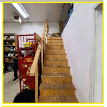
The photo above shows access stairs to the storage mezzanine. The stairs and railing are not built to code. A small unit heater is observed to be mounted to the underside of the ceiling in the gear room.
