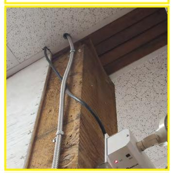
Reference previous photos for further information on photo above. This photo shows another partition wall. Exposed electrical and emergency lighting wiring is observed. The beam above is shimmed and appears to lack appropriate fastening requirement.
