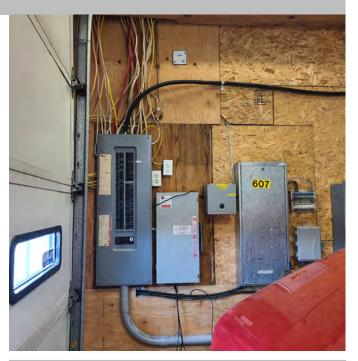
The photo above shows the surface mounted electrical room positioned within the apparatus bay area. This should be within a dedicated fire rated electrical room. The wiring and fuse switches are exposed and are very near to the door.
