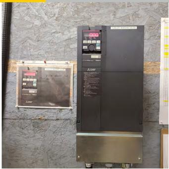
The photo above shows surface mounted equipment controls and surface mounted wiring again a painted OSB wall finish.
