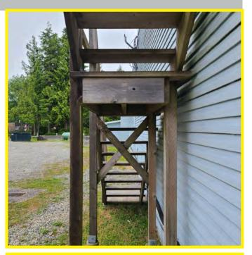
The photo above shows further evidence of the description to the right. The stairs are not properly secured to the building structure.
